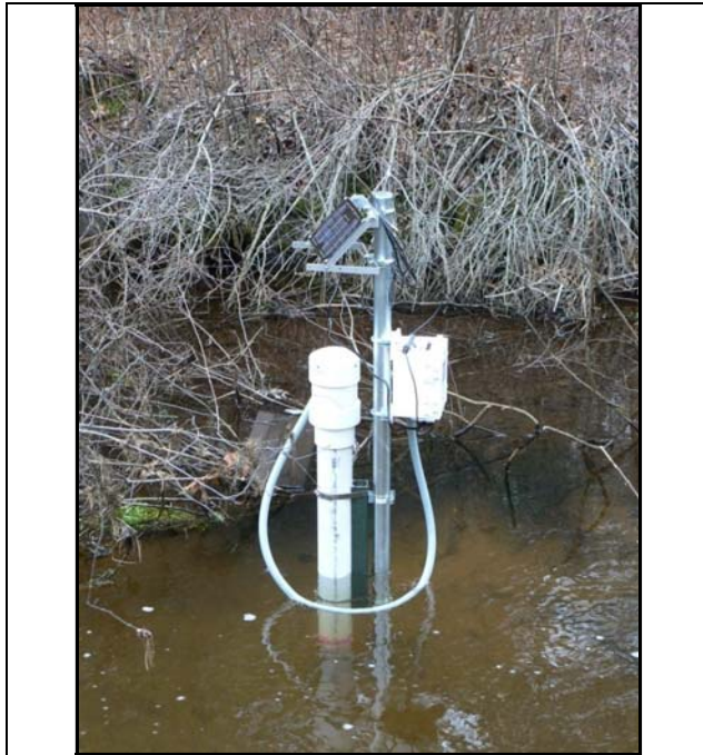
Figure 1: Remotely accessed water depth sensor installed at Red Brook with funding from this grant.
